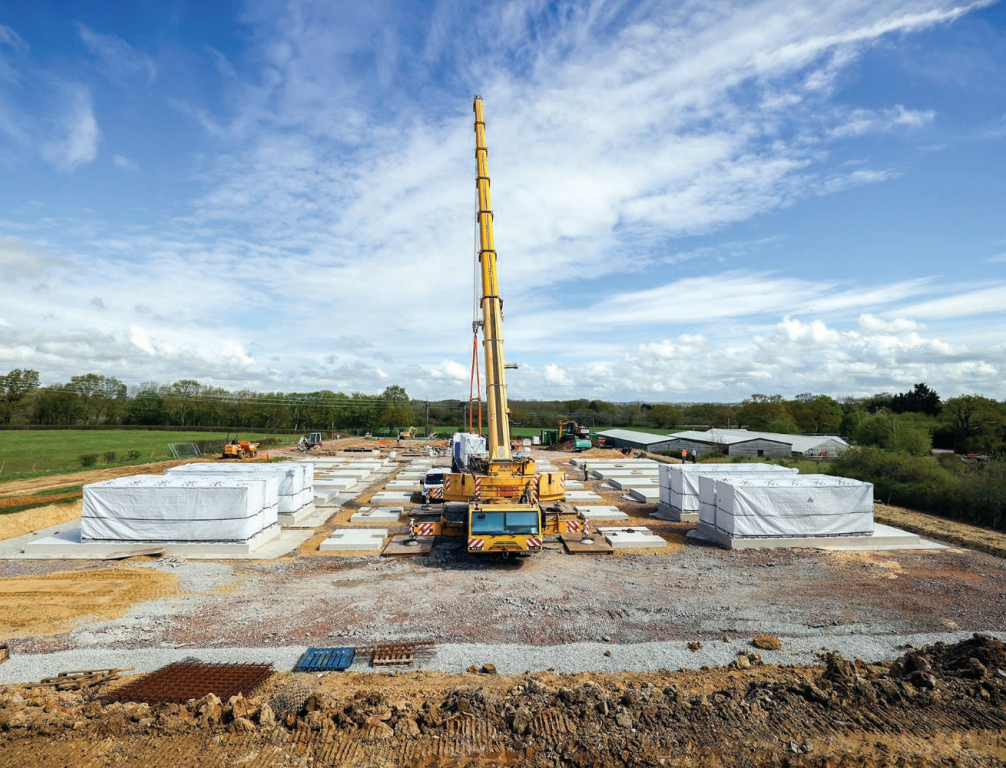
This energy storage facility under construction in southeast England uses lithium-ion batteries.
